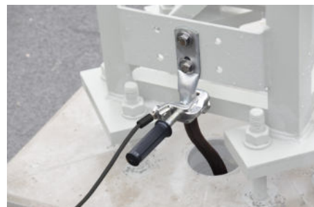
Earth connection with universal clamp
