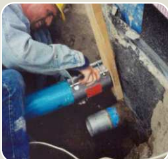
▲ U.S.: sewerage repair work
