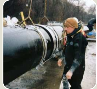
▲ UK: district heating work
