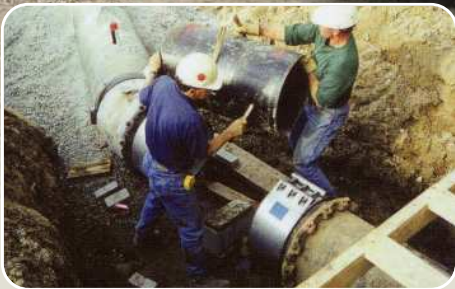
▲ Repair work for pipes replaced underground
